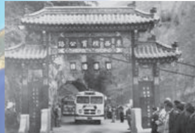
May 1960 marked the opening of the Central Cross-Island Highway
