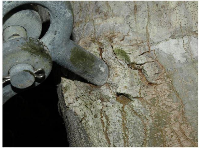
Fig 2. An eyebolt being overgrown by the tree
