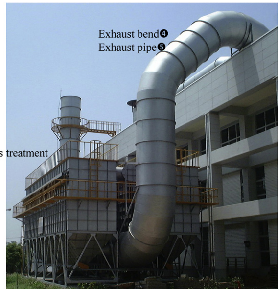
Fig. 2. Waste gas treatment system.
