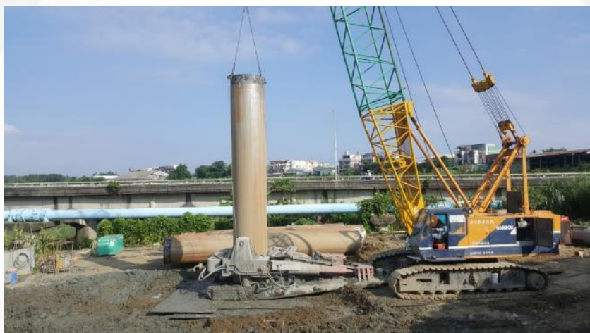
P4-全套管基樁鑽掘
