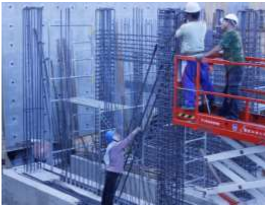
(c) 組裝對角向鋼筋
