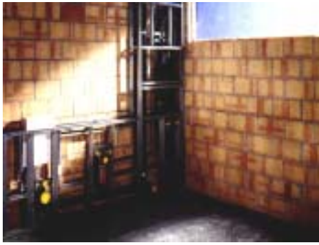
(a) 輕鋼架 + 矽酸鈣板
