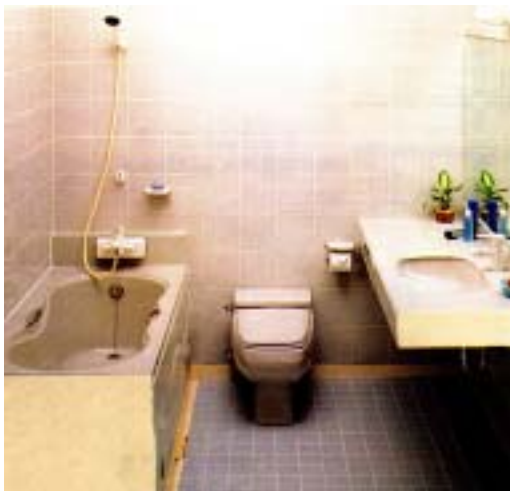
(a) FRP 牆版及底盤上貼磁磚
