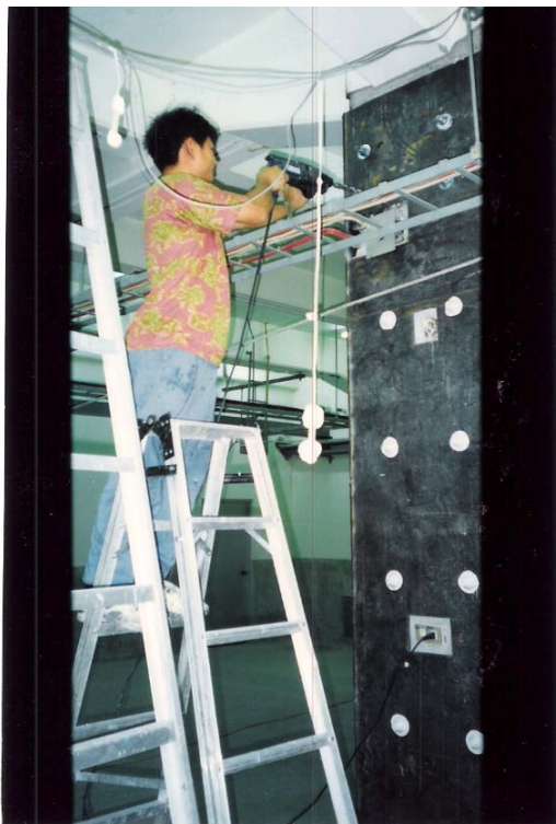
(c) 化學錨栓施工
