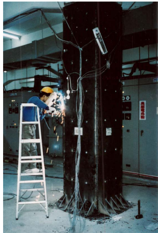
(b) 補強鋼板焊接
