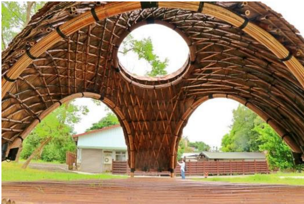
圖 5.25 共生-地景構造物之屋棚構造(取自 https://www.mysaiology.com/craftsman-news/article/taiwan-bamboo-architecture )
