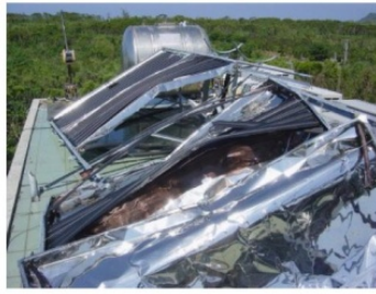
Figure 1.1.1 Damaged solar collectors (after Chung et al, 2008)
