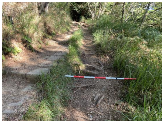
0.35K/鋪設路緣石22.5m 2
