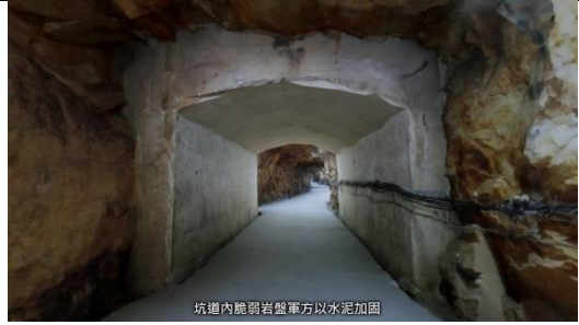
坑道內脆弱岩盤軍方以水泥加固
