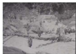
86.陶費溪(タフアイ溪)架設橋
