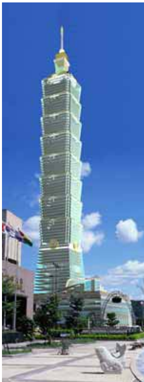
TAIPEI 101 BUILDING Taipei, Taiwan
