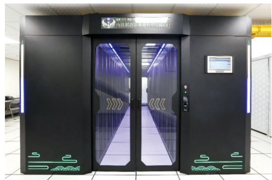
Hot and cold aisle closed system
